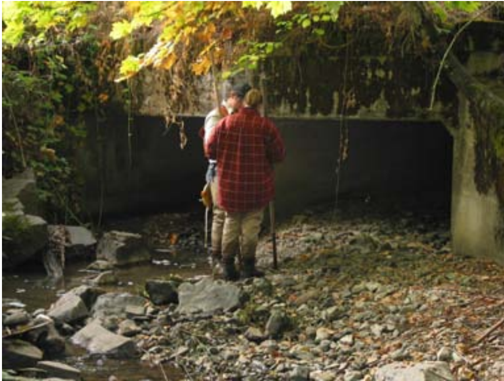
Figure 21. Culvert #1 outlet on Jordan Creek at I-5.
