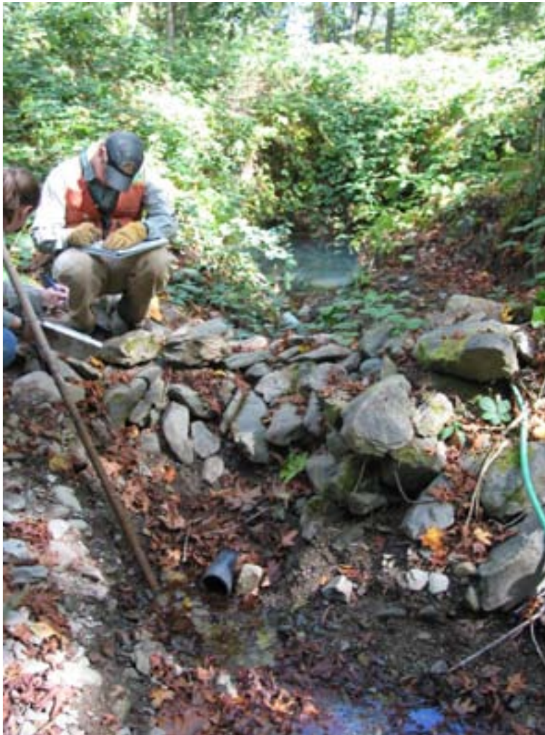
Figure 38. Water diversion on Alder Creek.
